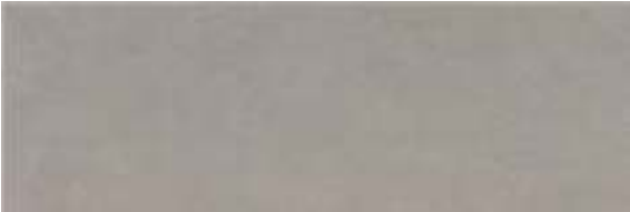
Wave Wall Concrete
