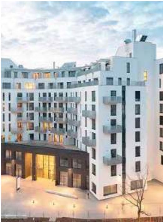
Althan Park Residential Complex | Austria
